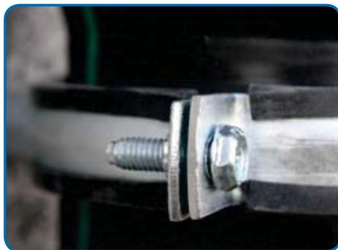
Figure 5 - Incorrect tightening:
